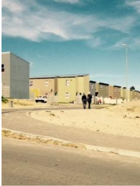
Newly built RDP houses (Photo: Avril Cowlin)
