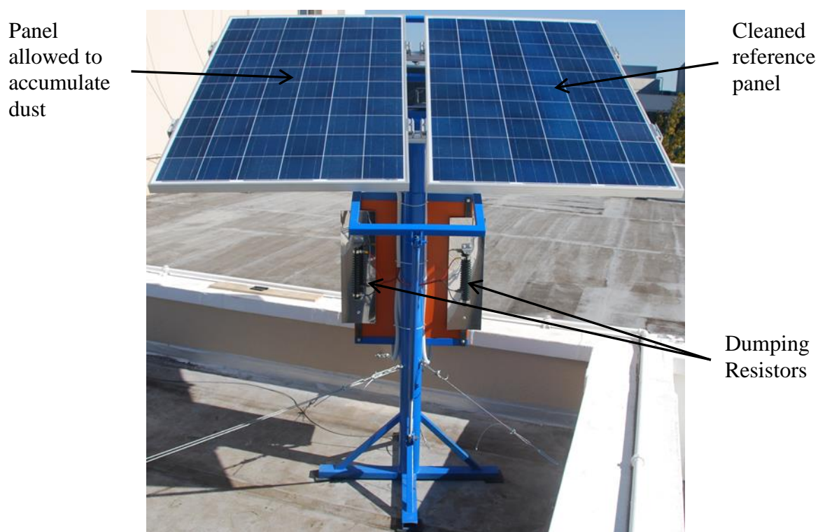
Figure 6-2: The picture of the station as mounted on the roof (Front View).
