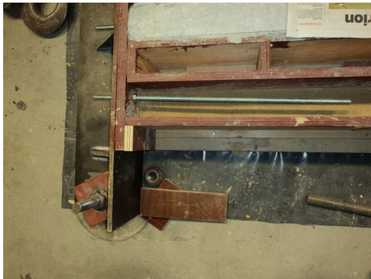
Figure 5.7: The threaded bar restraining the concrete against movement
