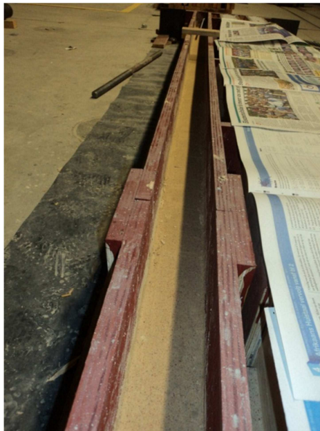
Figure 5.8: The compacted sand layer before casting
