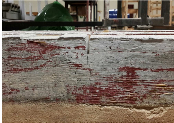
Figure 5.16: The crack at the joint
