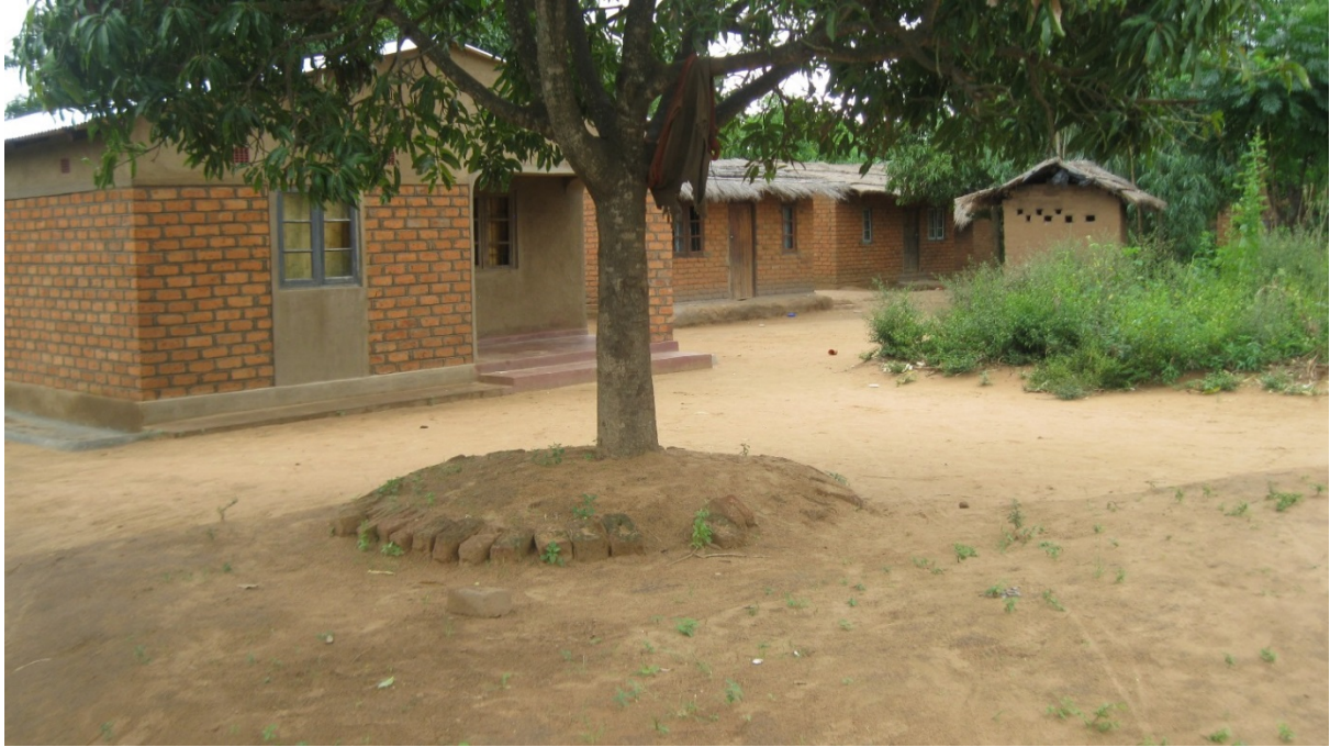
Figure 6: A brick house belonging to a better-off household (Photograph: B Matinga)
