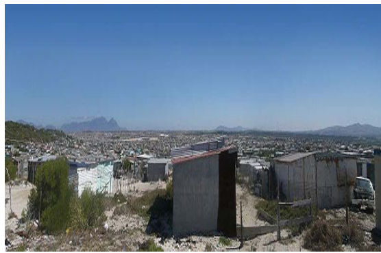
Fig. 2.7 Khayelitsha: close-up of ‘houses’ (21.10.2011)
