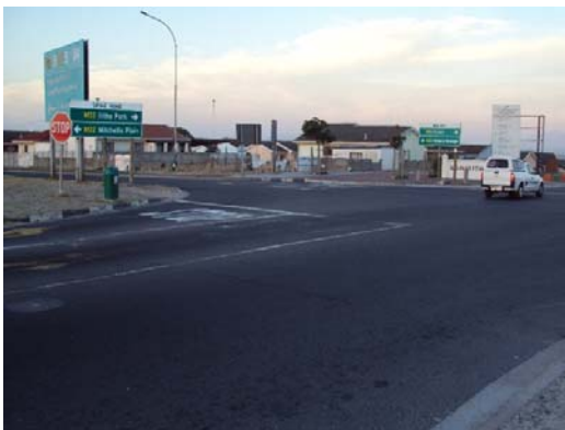
Figure 2.9 Mew Drive and Spine Road view (12.10.2011)
