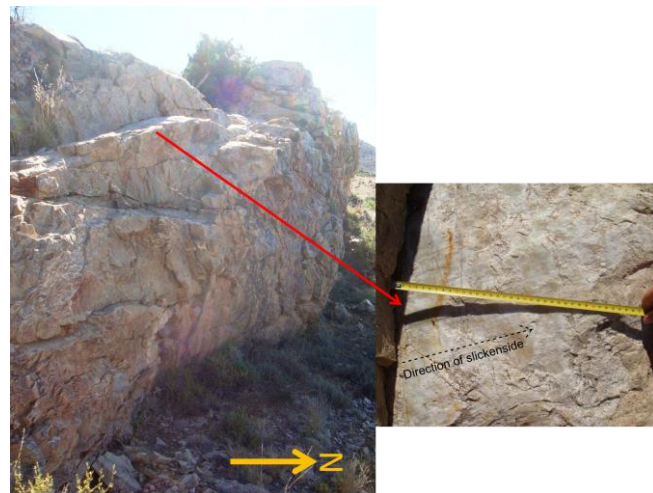
Figure 4.4: Outcrop of Sm at Miller showing veins and slickenside features on bedding.
