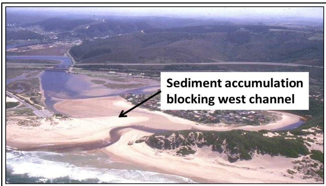
Figure 10: Sedimentation blocking the west channel ( www.dwaf.gov.za , accessed October 2014)
