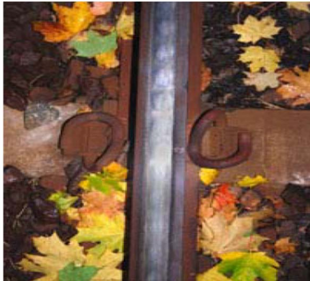
Figure 5-6: Rail Corrugation (Nielsen & Torstensson, 2010).
