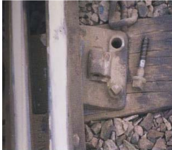
Figure 5-11: Timber Sleeper Failure (Hassankiadeh, 2011).
