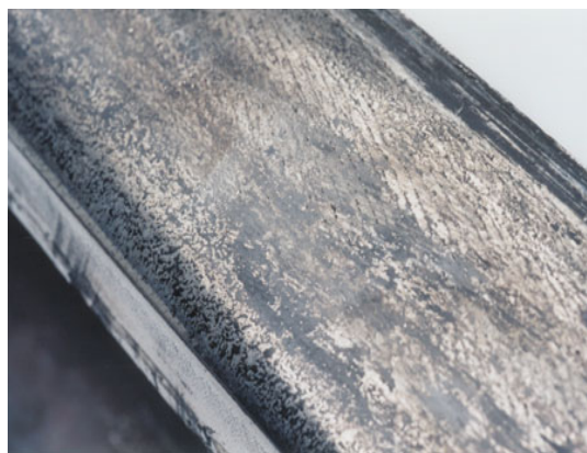
Figure 5-10: Head Check Defects (R06C0104, 2006).
