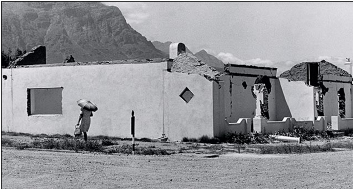
Figure 2.8: A heavily damaged masonry building in the Tulbagh (Thompson, 2012).
