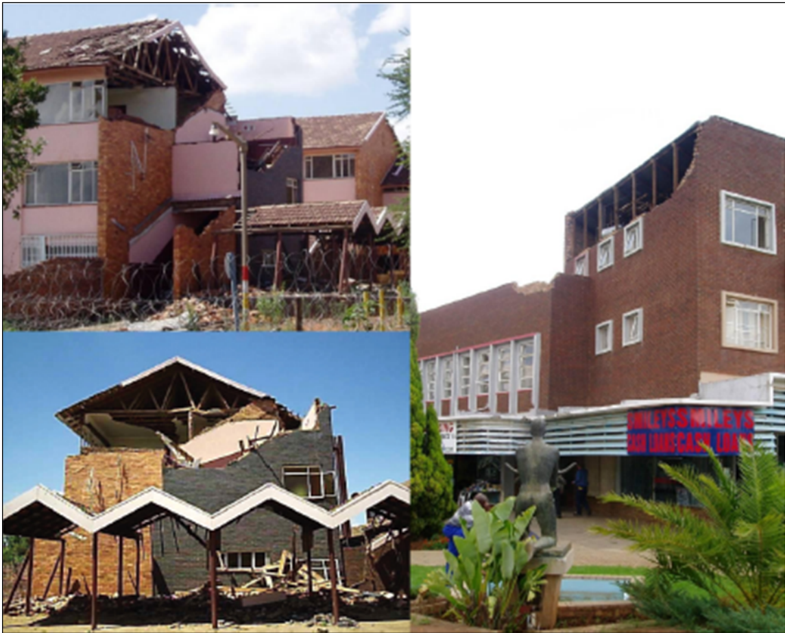
Figure 2.4: Damage to buildings after Stilfontein earthquake (Linzer et al. , 2007)
