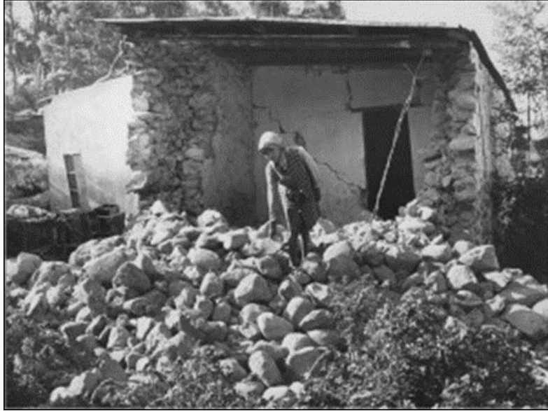
Figure 2.7: Damaged masonry building in the Tulbagh region. Note the natural construction materials that were used (Die Burger, 1989).
