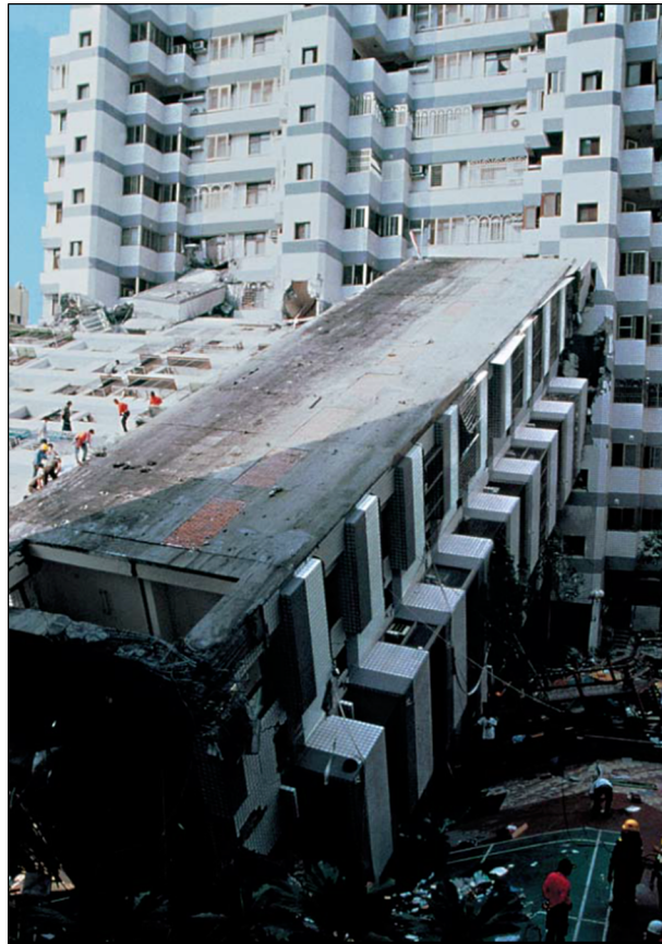
Figure 3.3: An overturned multi-storey residential building during the 1999 Taiwan earthquake (Bachmann, 2003)
