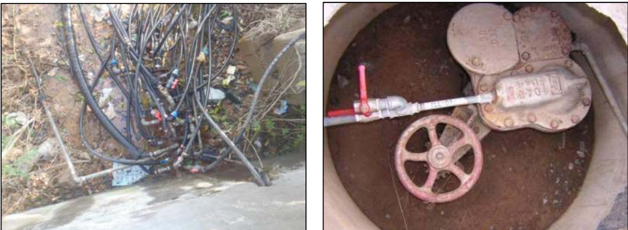
Figure 4.9: Examples of unauthorised connections on bulk water supply mains
