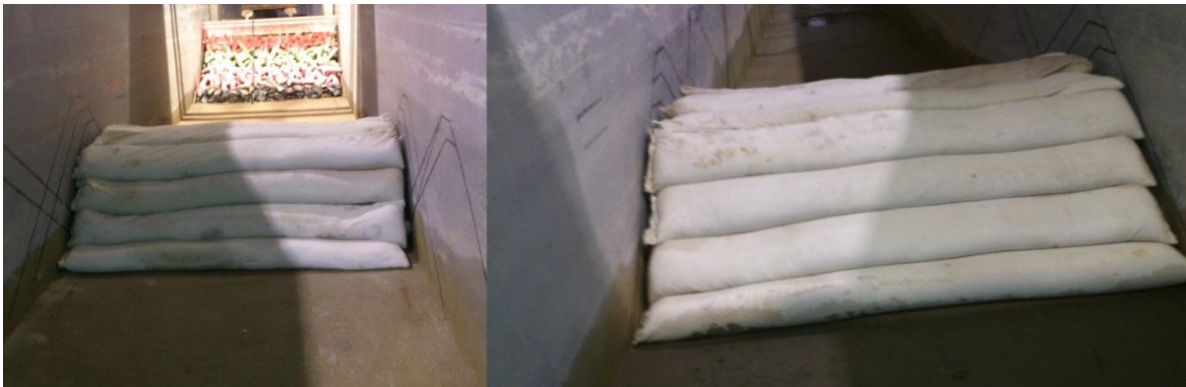
FIGURE 5.19: CONSTRUCTION OF GEOTUBE REEF BREAKWATER
