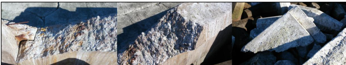
FIGURE 3.5: DAMAGED PORTIONS OF THE OVERTOPPING WALL AT VARIOUS POINTS ALONG THE BREAKWATER
