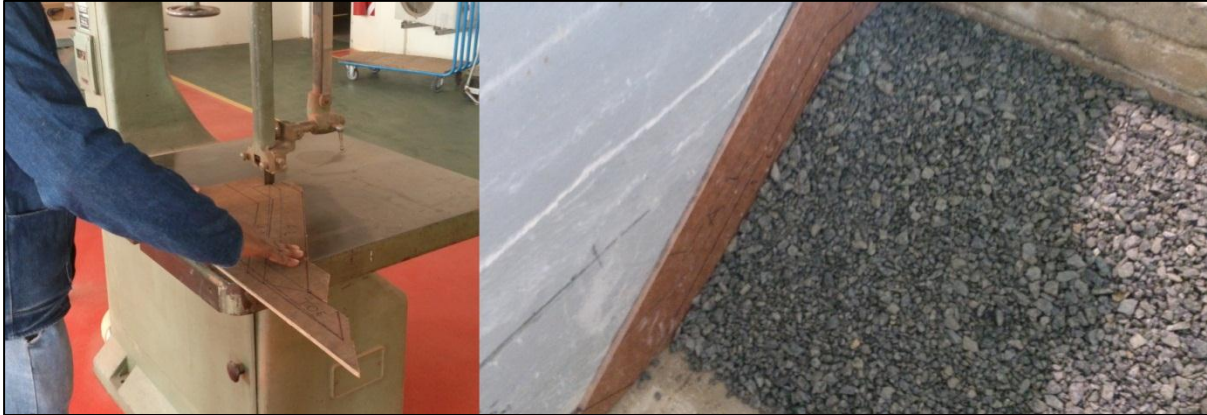
FIGURE C.1: CUTTING OF BREAKWATER TEMPLATES (LEFT) AND CORE CONSTRUCTION (RIGHT)
