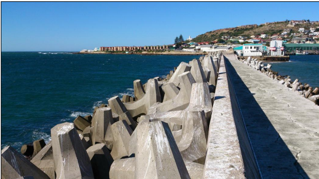
FIGURE 3.4: VIEW ALONG MOSSEL BAY BREAKWATER (LOOKING SOUTH-EAST)
