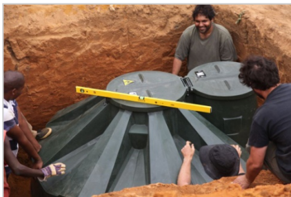
Figure A 7. Biogas digester
