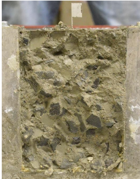
Figure 9.7: Fully cracked surface area of a 5h test specimen
