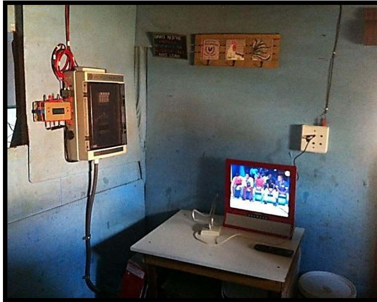
Figure 13: Solar system – Enkanini (picture)
