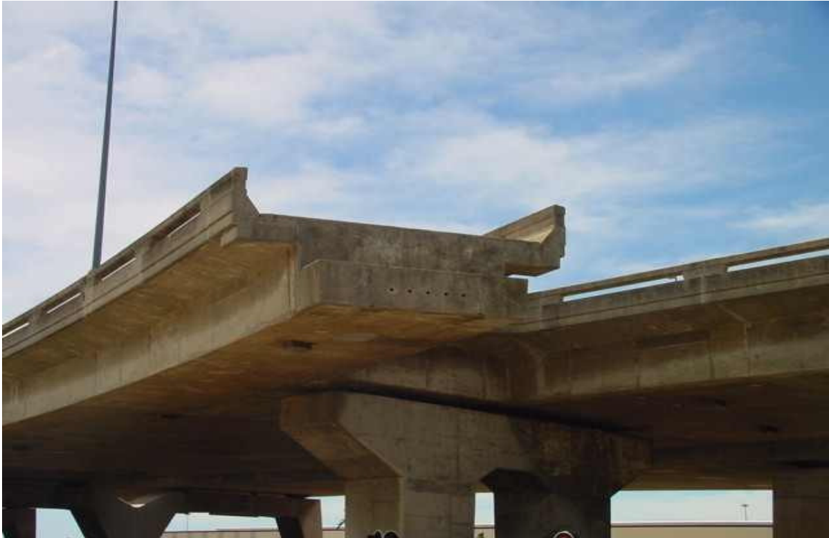
FIGURE 1.2: BAAKENS PARKWAY RAMP STUB
