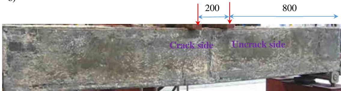
Figure 7-6: Box girder 1: (a) Force deflection curve; and (b) Crack opening photo.
