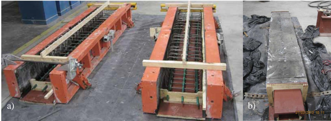
Figure 7-3: Post tensioned box girder: (a) before casting; and (b) after de-moulding.
