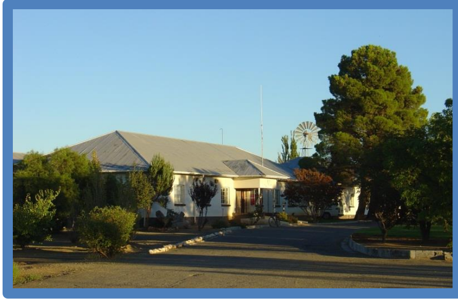
Figure 6.10. The Community Health Care Centre at Fraserburg
