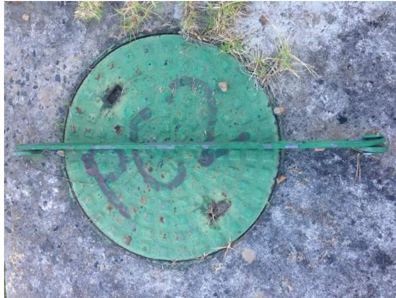
FIGURE 4.2: Manhole with lock system in place, Botmaskop reservoir October 2014.
