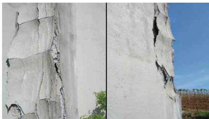
FIGURE 5.5: Deterioration caused by sulphate attack [MAPEI, 2011].
