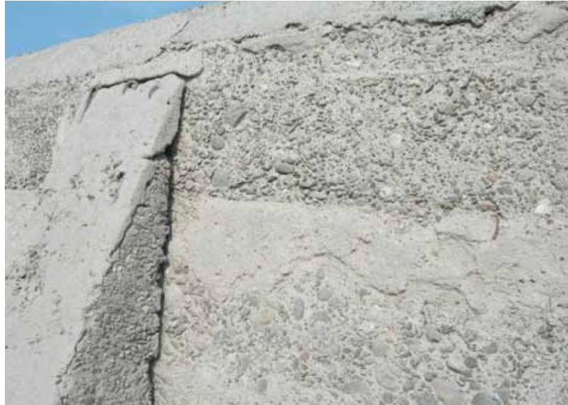
FIGURE 5.3: The Effect of Leaching on a Concrete Surface [MAPEI, 2011].
