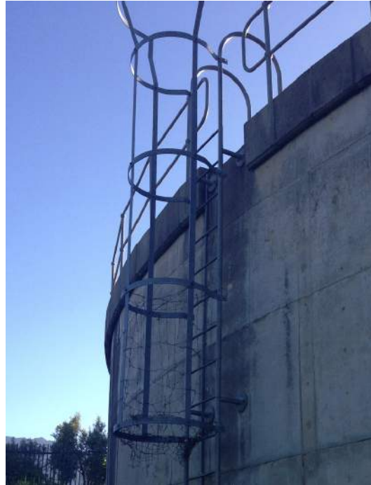
FIGURE 4.1: External Access Ladder with vandalism damage to ladder door, Botmaskop reservoir October 2014.
