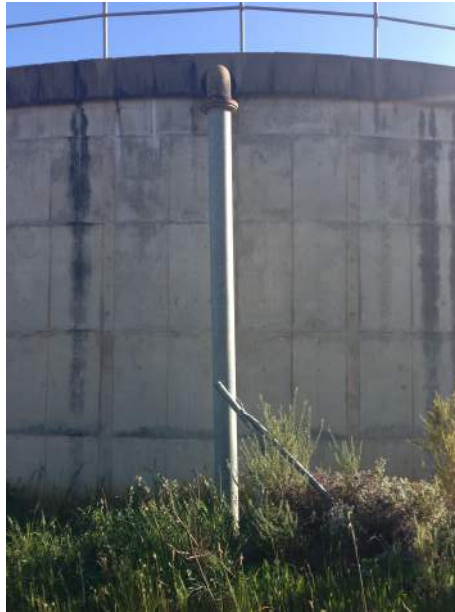
FIGURE 4.5: Reservoir Overflow pipe, Botmaskop reservoir October 2014.
