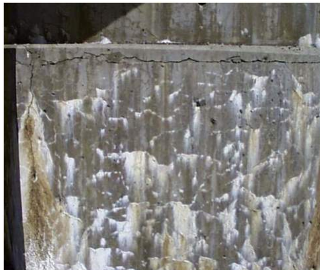
FIGURE 5.10: White Deposits from ASR [Farny and Kerkhoff, 2007].
