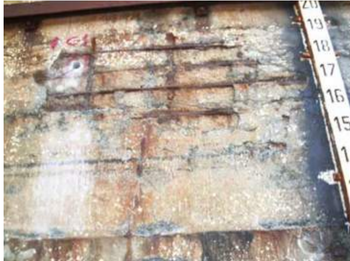
FIGURE 5.6: Reinforcement corrosion due to chloride ingress with secondary concrete delaminations [MAPEI, 2011].
