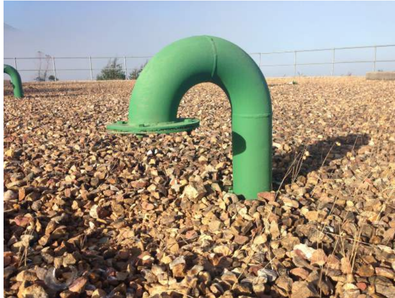
FIGURE 4.3: Reservoir Ventilator consisting of two 90^\circ bends with mesh, Bot-maskop reservoir October 2014.
