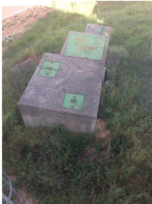
FIGURE 4.4: Drainage sump situated nearby to reservoir, Botmaskop reservoir October 2014.
