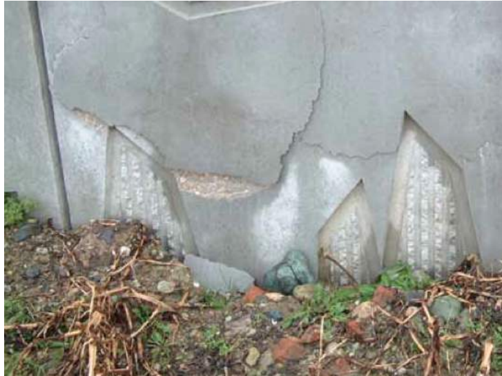
FIGURE 5.12: Deterioration caused by Frost Action [MAPEI, 2011].
