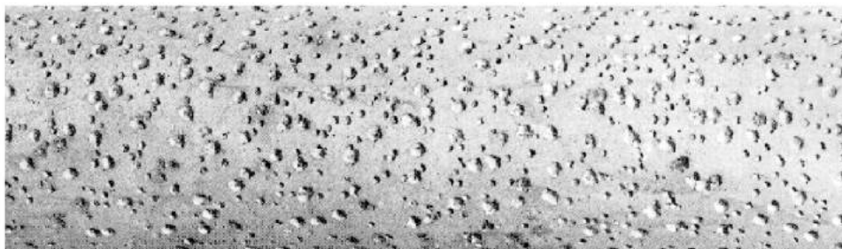
FIGURE D-7: Pitting of Piping section [Schmutz, 2013].
