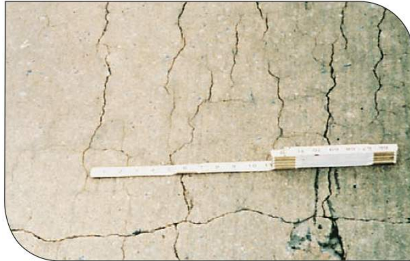
FIGURE 5.9: Longitudinal Cracks as a result of ASR [Farny and Kerkhoff, 2007].
