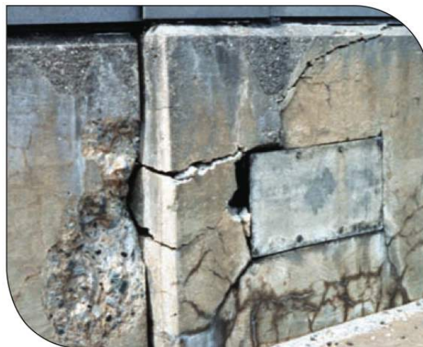
FIGURE 5.8: Severe Deterioration caused by ASR. Visible cracking, joint closing, spalling of concrete, lateral offset of concrete [Farny and Kerkhoff, 2007].
