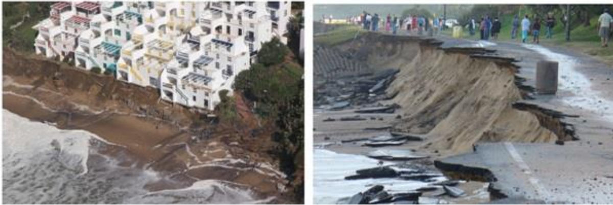
FIGURE 1. 5 - STORM WAVE DAMAGE IN KZN (MATHER ET AL 2011)
