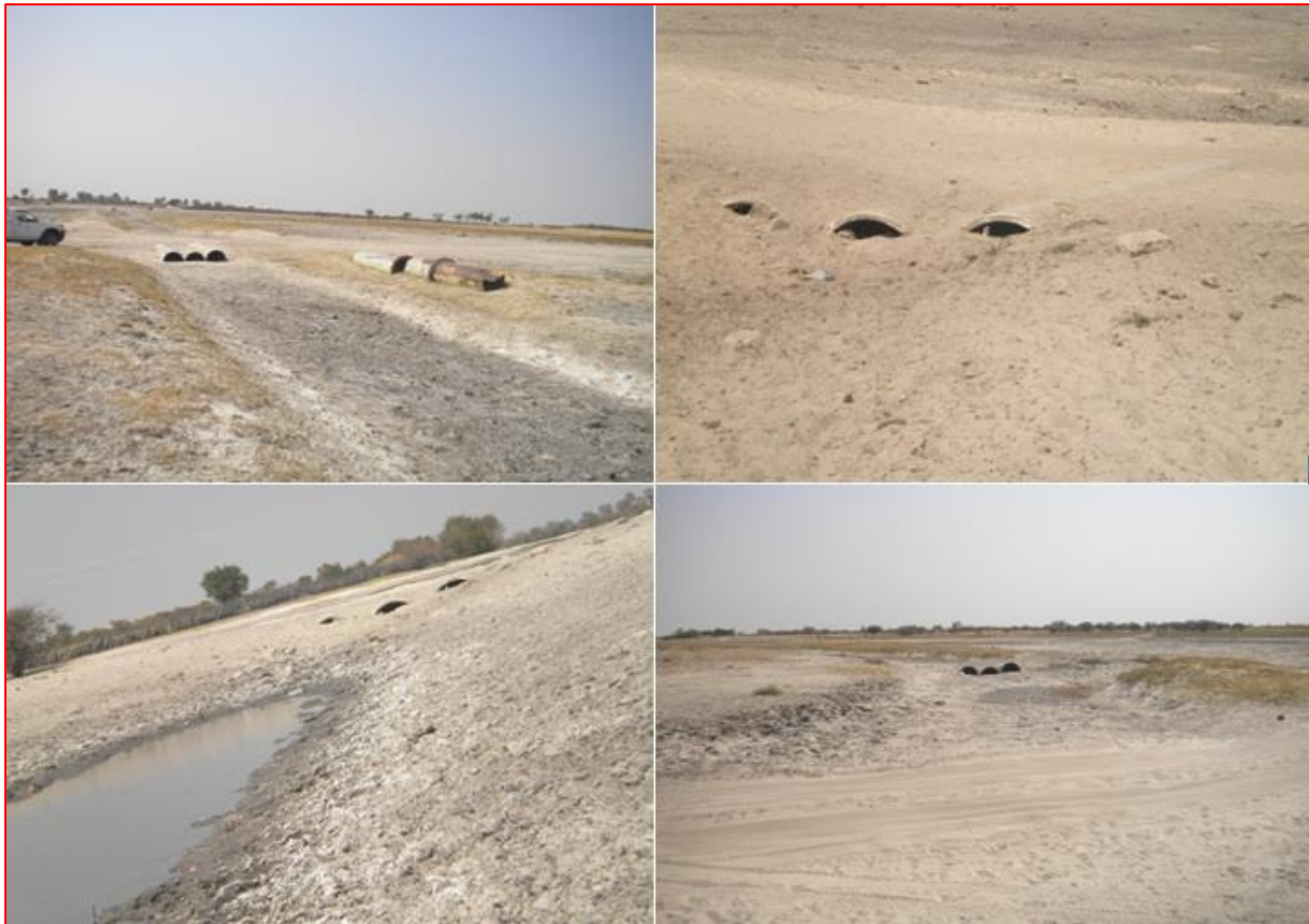
Figure 5. 23 Some of the inappropriate sand choked culverts in iishana channels
