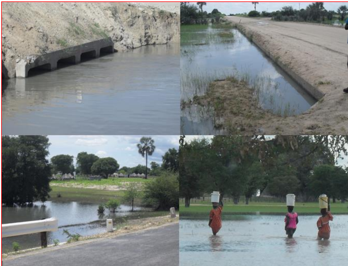
Figure 7. 1 Flooding due to smaller than necessary culverts and inappropriate construction during the 2013/2014 flood season
