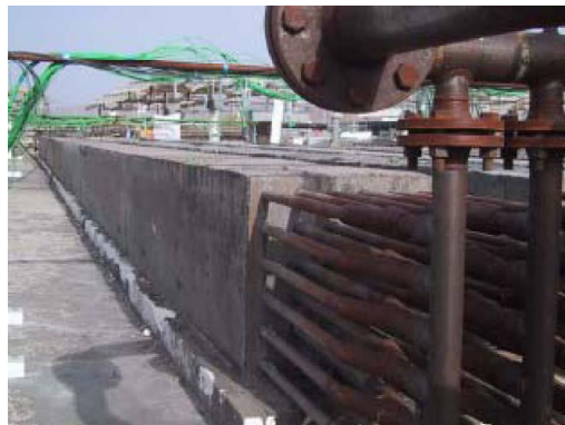
Figure 9 - Concrete storage with heat exchanger pipes visible at the end (Tamme, 2007)
