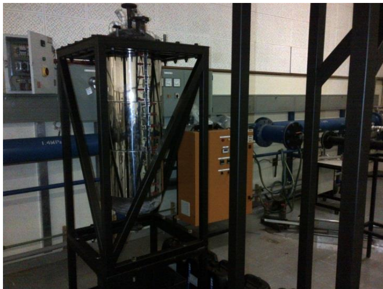
Figure 50 – Band heaters installed around the storage vessel
