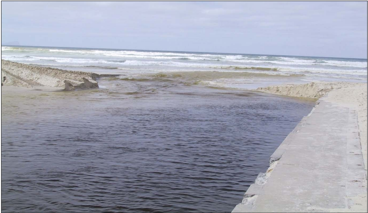
Figure 26: Mechanical opening of Zandvlei estuary mouth (City of Cape Town Municipality, 2008)
