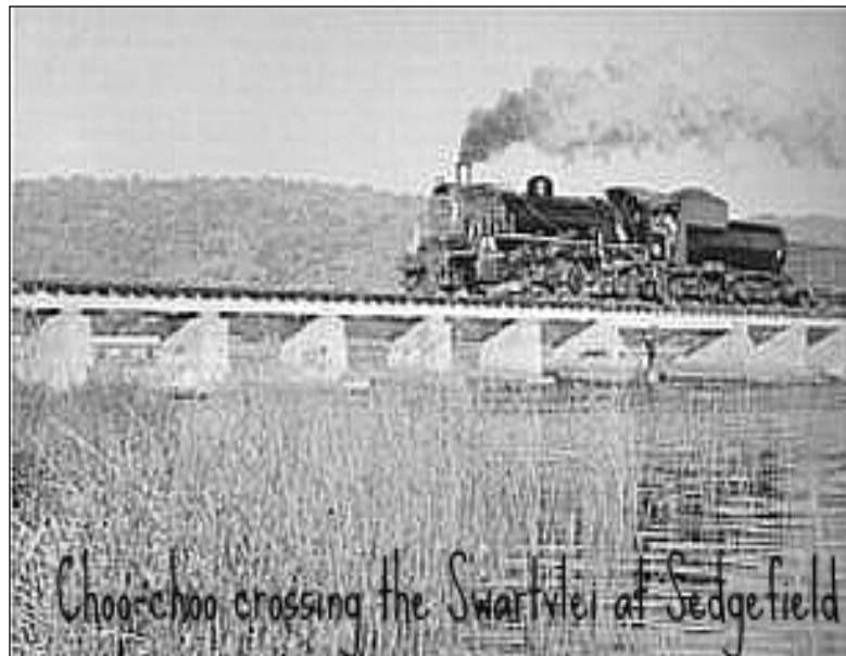
Figure 28: Railway crossing over Swartvlei
