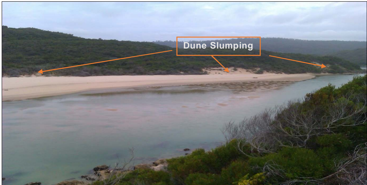
Figure 87: Western bank of estuary with slumping present
