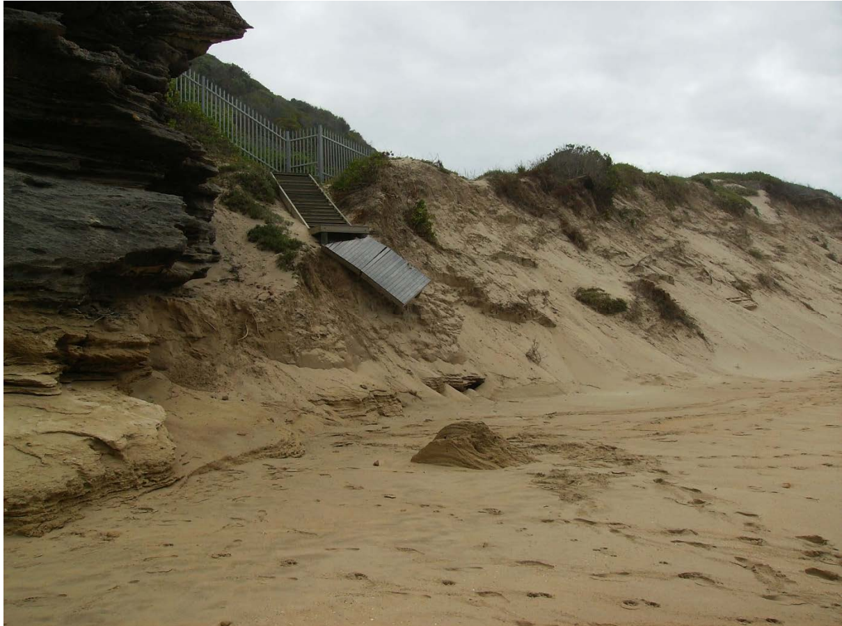
Figure 135: Erosion at profile seven
