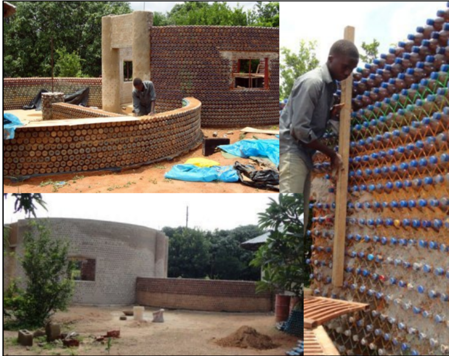
Figure 2.8: Plastic bottle house construction (Olukoya, 2011)
