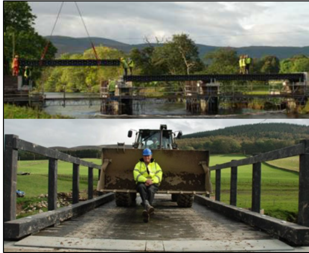
Figure 2.10: Vertech material bridge. First thermoplastic bridge in the UK (Vertech, [S.a])
