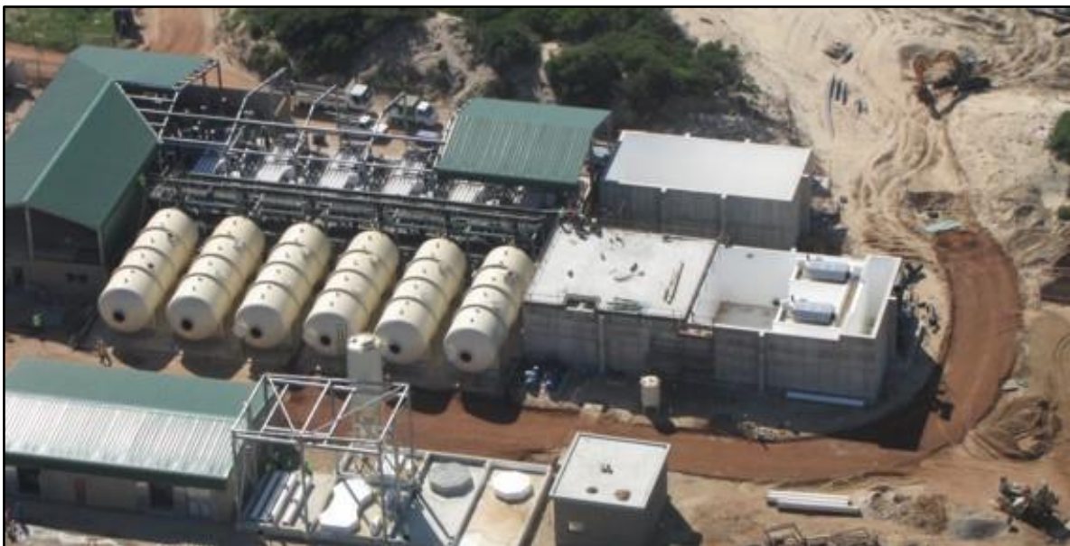
Figure 3.1: Mossel Bay desalination plant (Mossel Bay Municipality, 2011)
