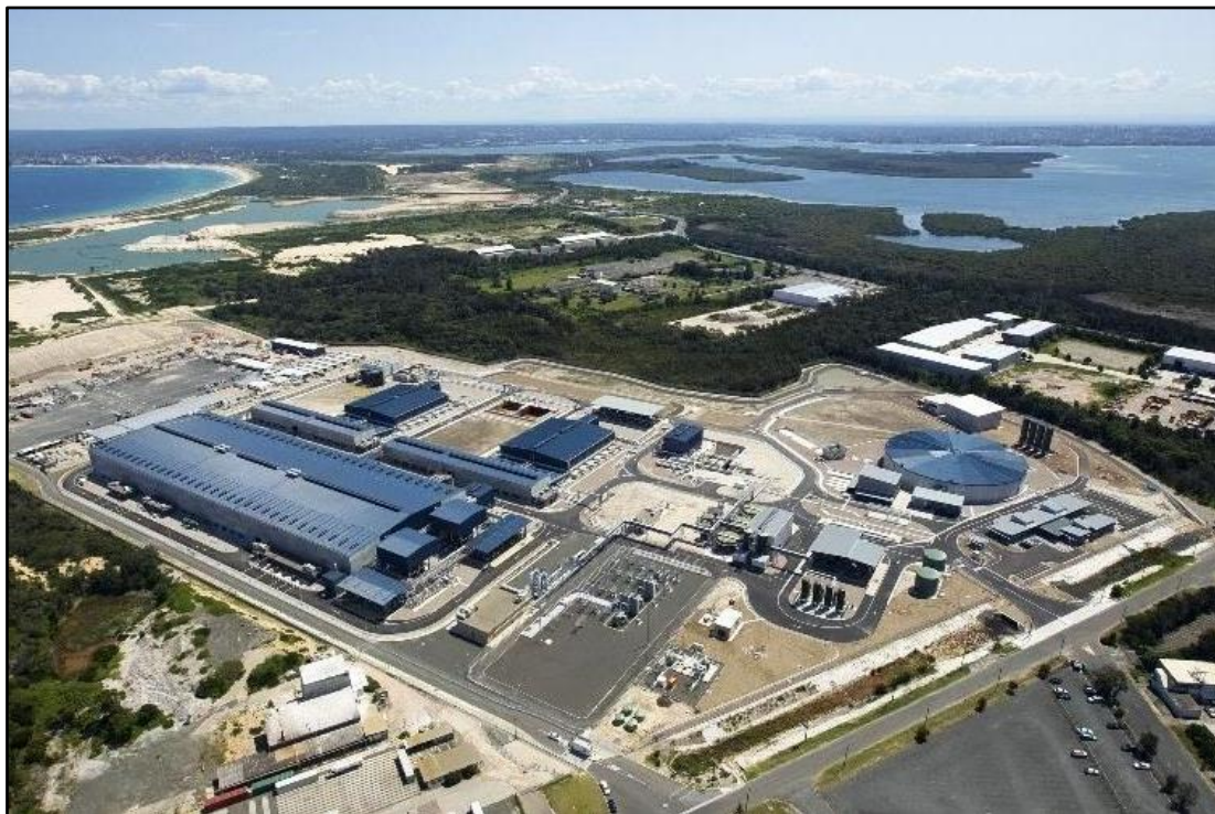
Figure 3.5: Aerial view of Kurnell Desalination Plant (La Perouse, 2010)
