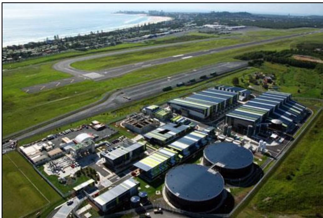
Figure 3.6: Tugun (Gold Coast) Desalination Plant (Water Technology, 2011)
