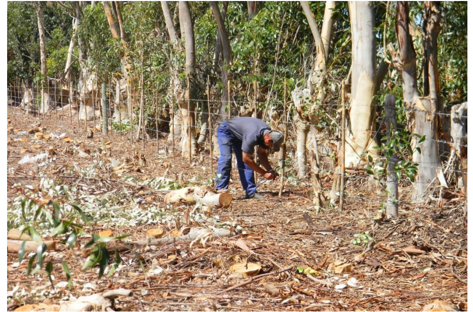
Image 3.2: Droppers being used in the erection of fences (Credit: Carlo Cloete).
