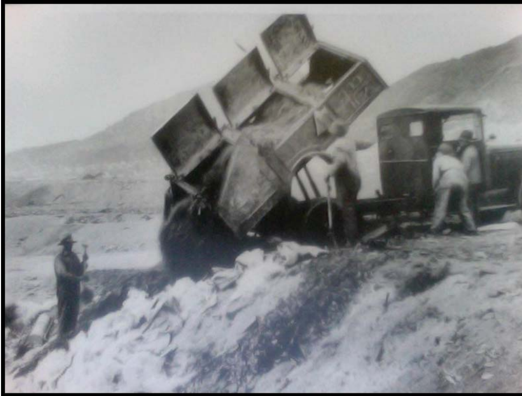
Figure 5: City Council Tip-Truck No. 11 tipping refuse at Three Anchor Bay 246
