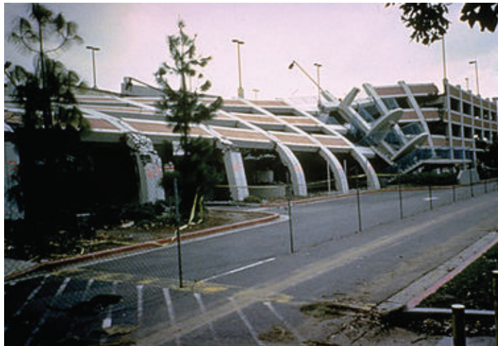
Figure 1.3: The Failure of a California State University Structure in 1994
