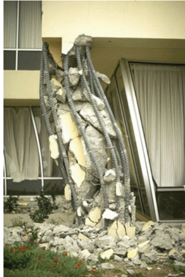
Figure 1.2: The Failure of a Column at Olive View Hospital in 1971
