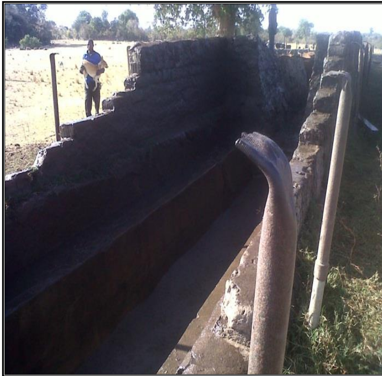
Figure 3.1: Mavhaire Dip Tank, Buhera, Manicaland
