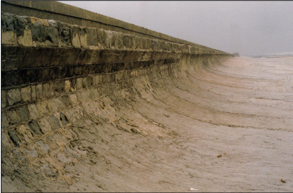
Figure 22: Recurve seawall near Dymchurch, United Kingdom
