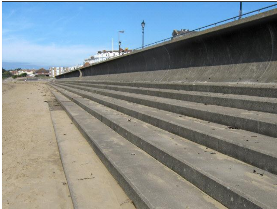
Figure 19: Stepped seawall with recurve at Burnham-on-Sea, Somerset, United Kingdom
