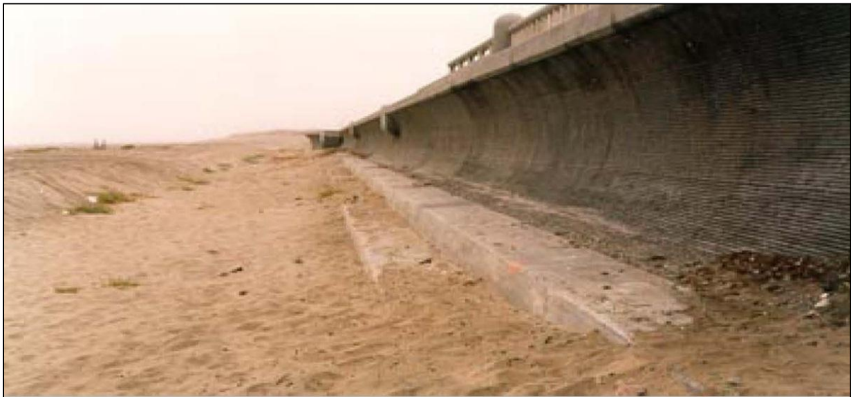
Figure 25: Recurve seawall at Ocean Beach, San Francisco, CA, USA (Noble Consultants, Inc., 2011)
