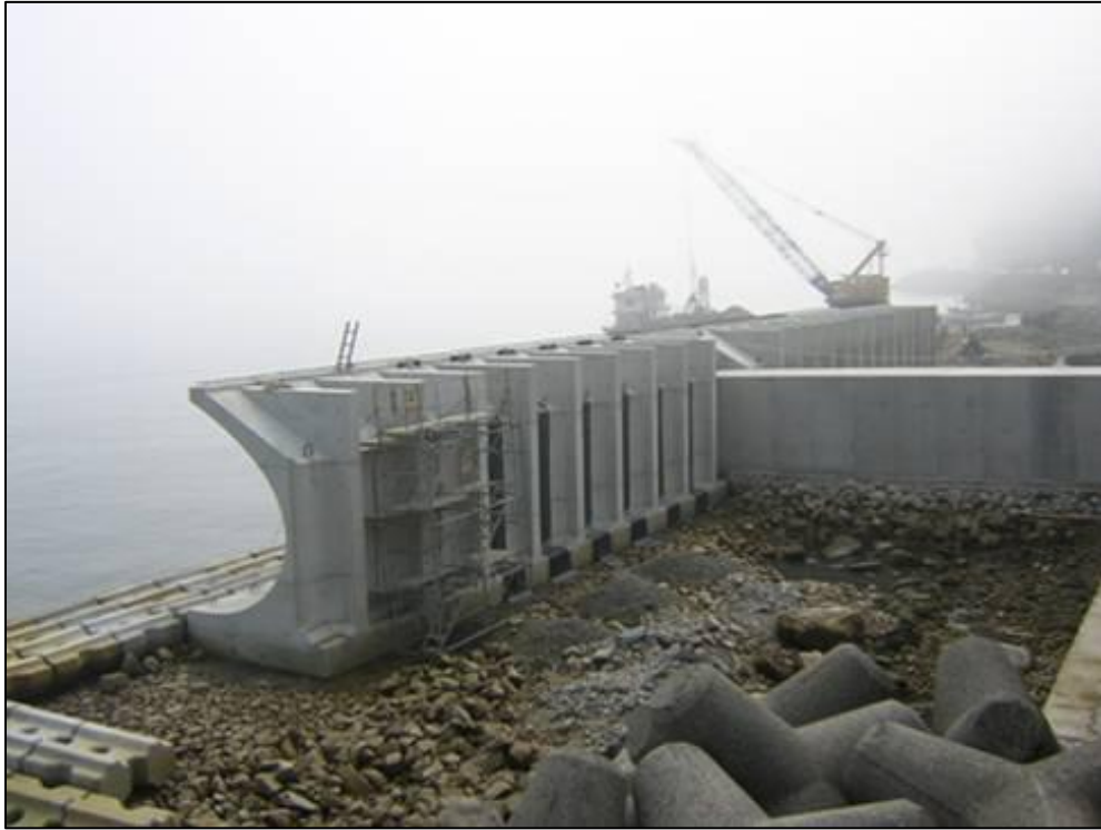
Figure 26: Construction of the Flaring Shaped Seawall (FSS) in Kurahashi-jima, Hiroshima, Japan (Kamikubo, n.d.)
