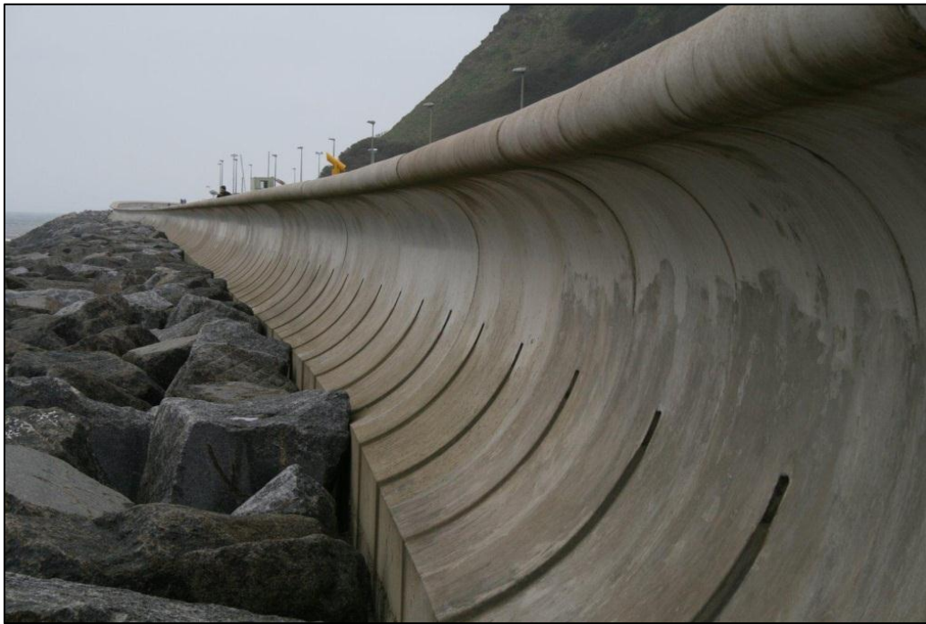
Figure 21: Recurve seawall with rock armour at Scarborough, United Kingdom
