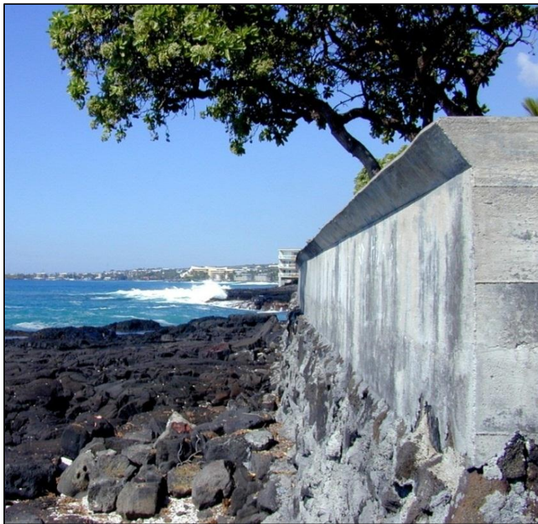
Figure 23: Recurve seawall at Kailua-Kona, Hawaii
