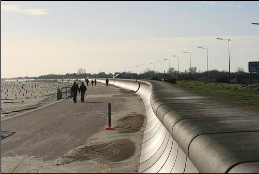
Figure 20: Seawall at St. Mary's Bay, United Kingdom
