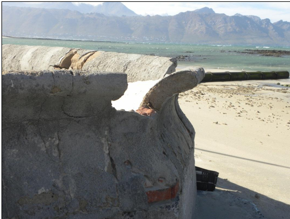
Figure 29: Damaged recurve wall in Strand, South Africa
