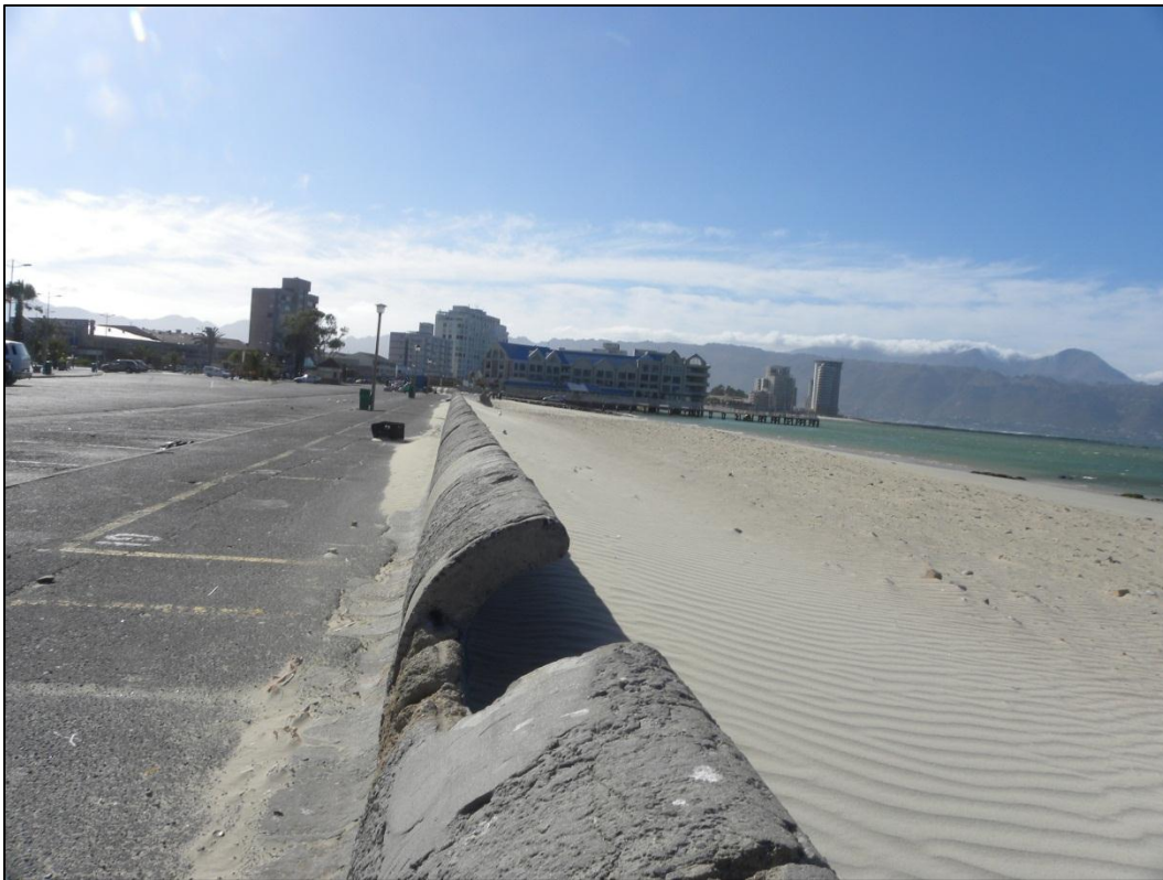
Figure 60: Current recurve wall in Strand
