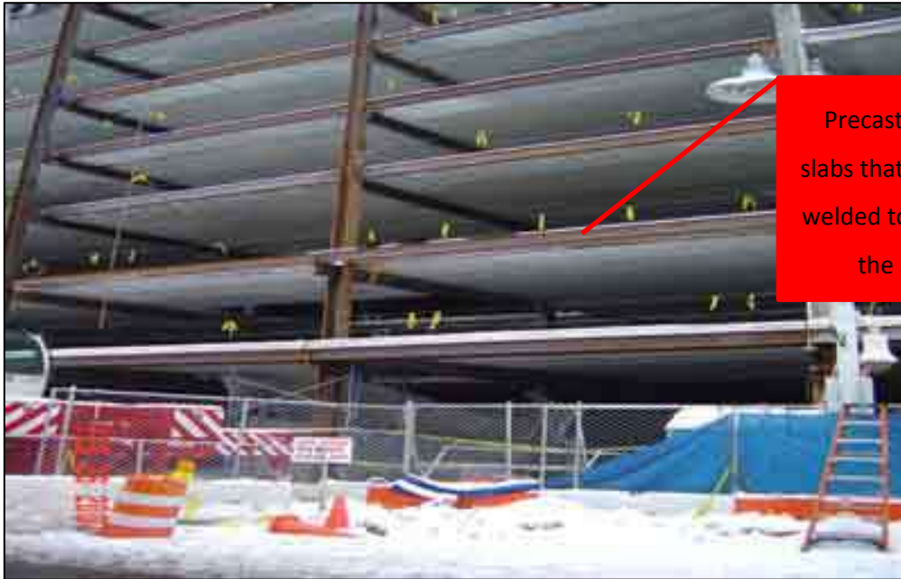
Figure 7: The steel framework and the concrete members that were placed on the steel beams (Higgins, 2004)
