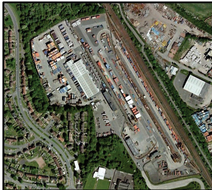
Figure 63: Layout of Coatbridge Freightliner Terminal (IBI Group, 2006)
