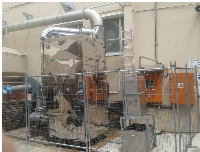
Figure K.4: Sauna diesel tank and measuring and control equipment view
