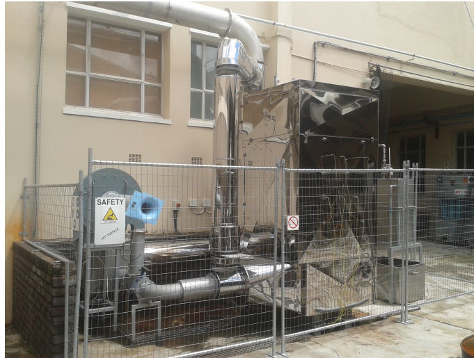
Figure K.3: Sauna diesel burner and blower view
