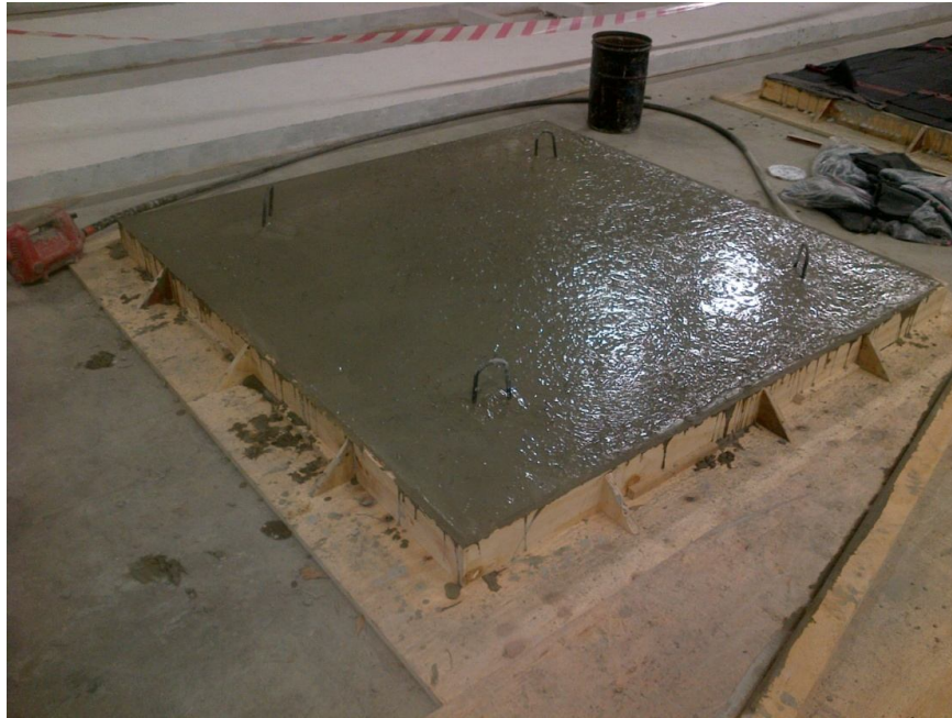
Figure 6.1: A SynFRC slab on the day of casting.
