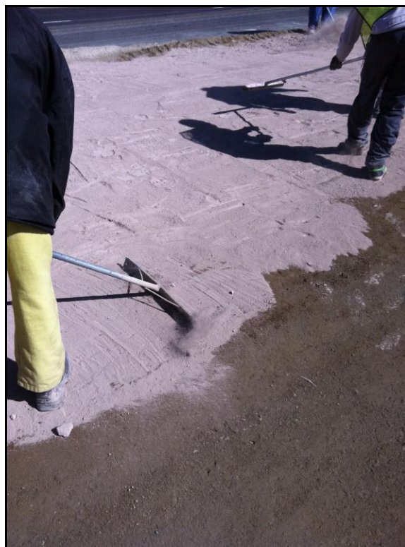
Figure 4.10: Spreading of cement or lime before in-situ recycling.
