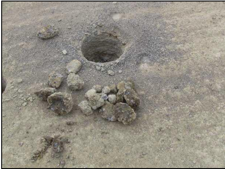
Figure 4.7: Broken-down cement stabilised granular material (Theyse 2013)
