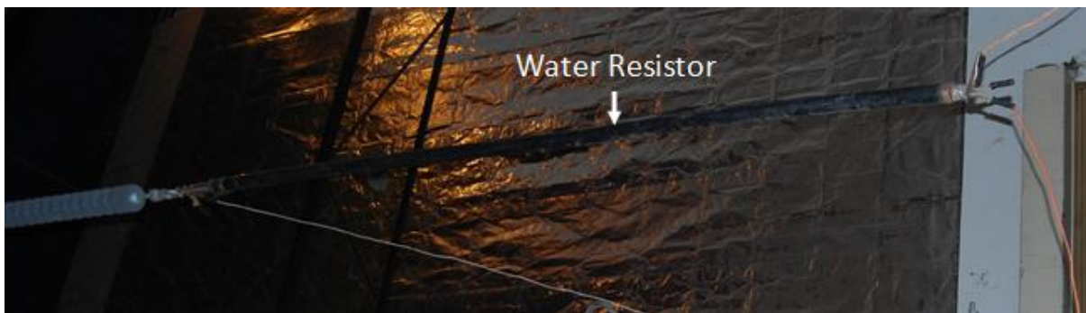
Figure 3.20: The water resistor, R_1 , suspended in the HV lab.
