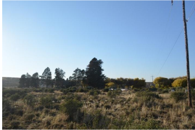
Figure 5.2: The trees close to the transformer as seen from the spark gap position.
