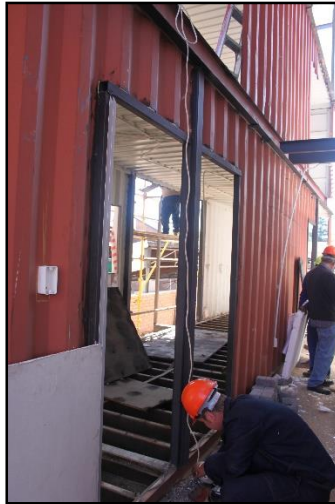
Figure 4.1 - On-site manufacturing of ISBU residential building (M. Hart, 2013).
