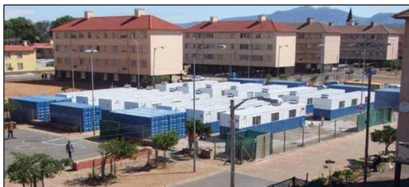
Figure 5.2 - Temporary container village (Keuler, 2013).
