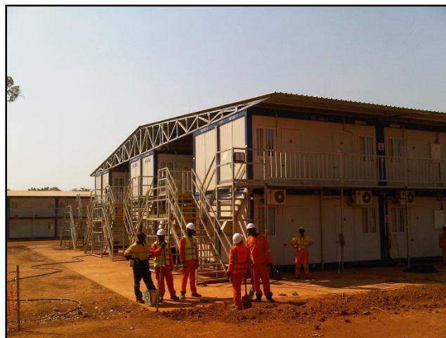
Figure 4.2 - Spaced container design for offices (FSM, 2013).
