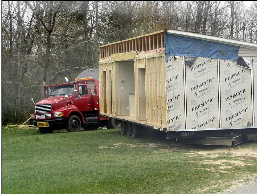
Figure 2.6 - A mobile home partway under construction (Melton, 2008).
