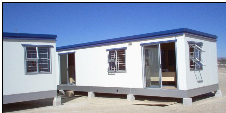
Figure 2.5 - A manufactured house (Fabricated Steel Manufacturing, 2013).
