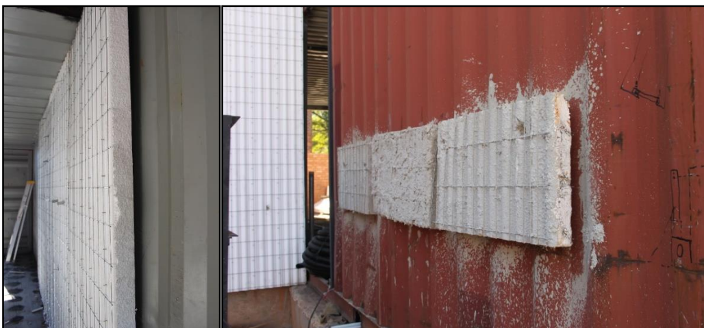
Figure 4.15 - EPS sheets with wire mesh, and applied shotcrete-type coating.
