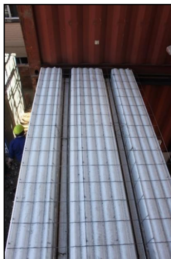
Figure 4.14 - EPS slab permanent formwork system.
