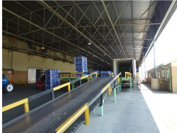
Figure 13: Loading area covered only by a sink roof
