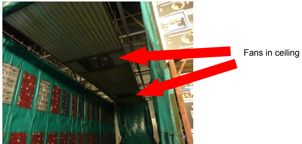
Figure 8: Empty forced-air cooling tunnel
