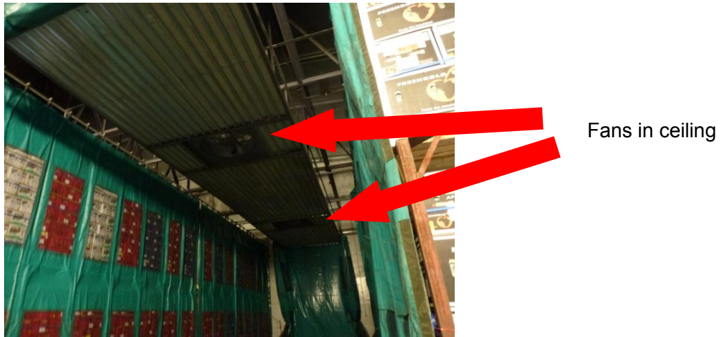
Figure 4.9: Empty forced-air cooling tunnel
