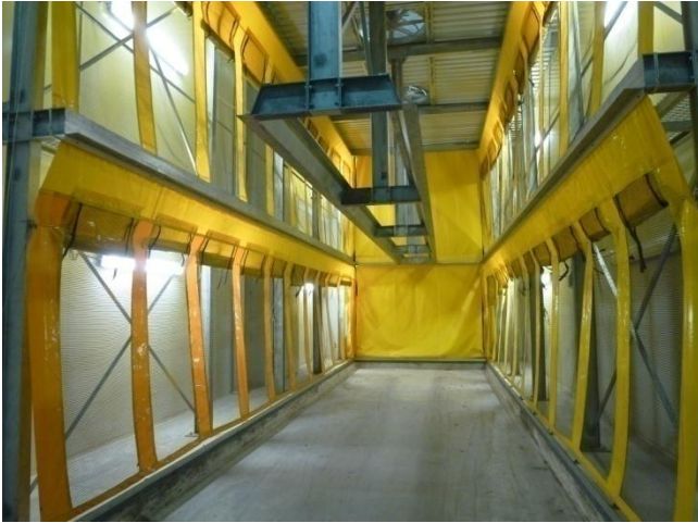
19: Forced air cooling tunnels inside cold store
