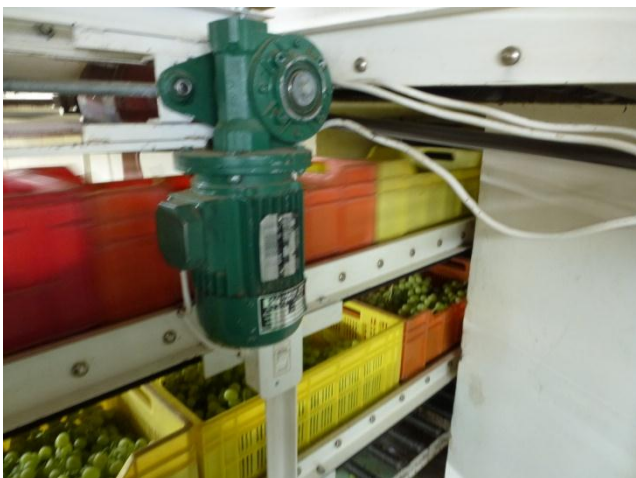
5: Grapes entering the pack house via a conveyer belt from the pre-cooling unit
