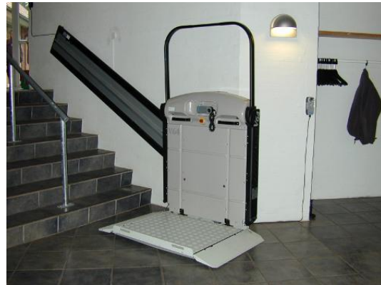
Figure 2: Public Stairlift Platform
