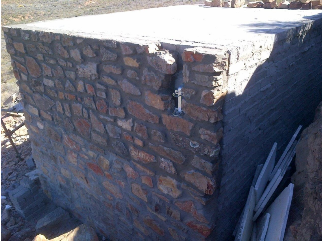
Figure C.11: Bracket for the communications pole/antenna.
