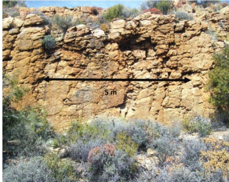
Figure 2.18: Rock face into which vault was to be constructed, with a 5 m imaginary core (Croukamp et al. , 2011).
