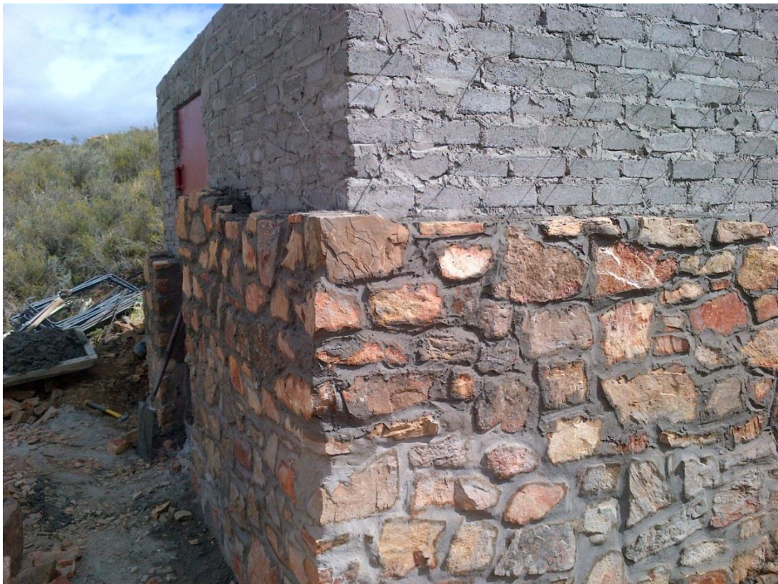
Figure C.6: Stone cladding on the sides of the walls.
