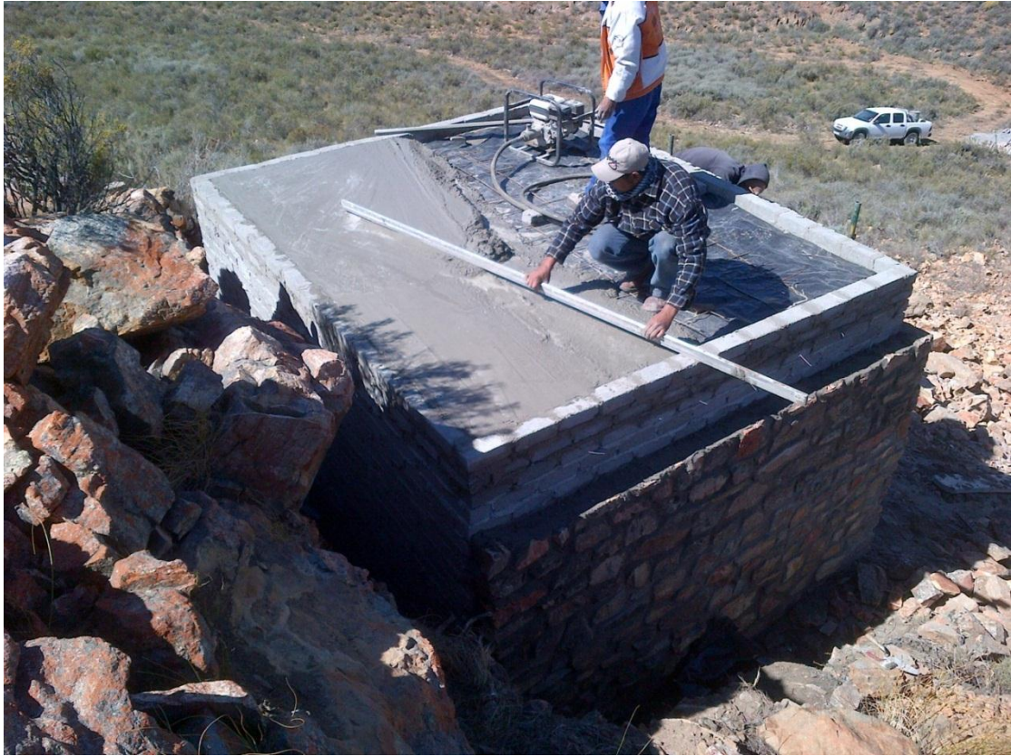
Figure C.9: Concrete slab on the top of the roof with plastic to prevent seepage.
