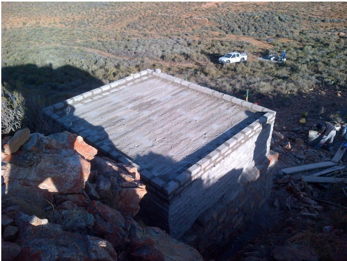
Figure C.8: Roof of lintels stacked next to each other.
