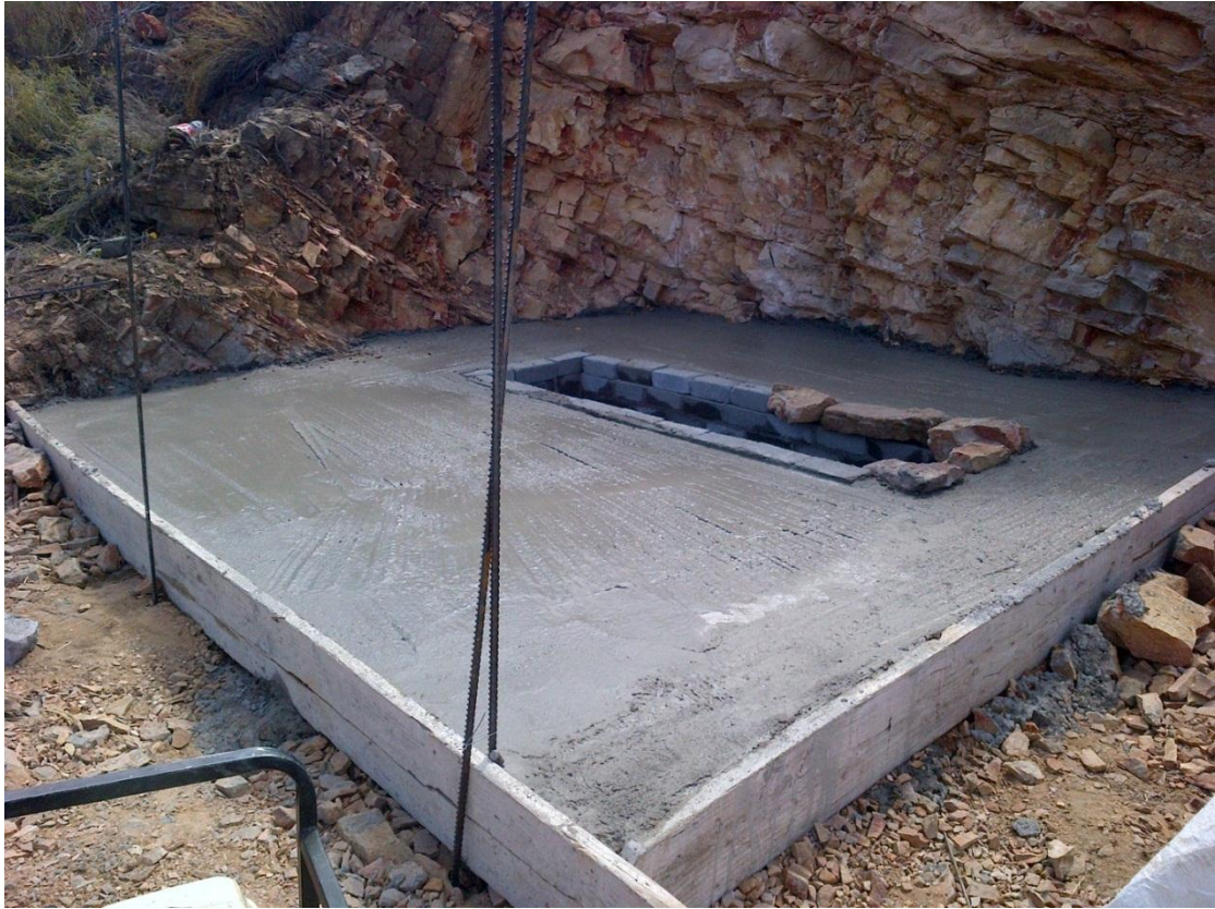
Figure C.3: Foundation at completion.
