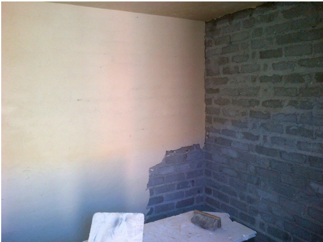
Figure C.10: Inside walls and ceiling plastered with cretstone.
