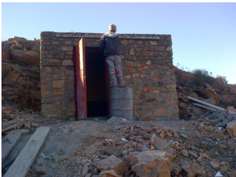
Figure 4.9: MGO gravimeter vault at completion.
