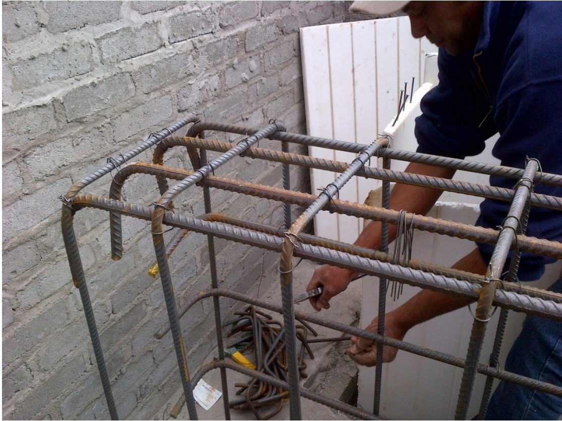
Figure C.7: Installation of plinth reinforcement.
