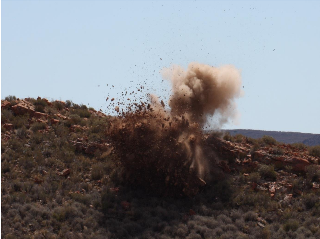
Figure C.1: Blasting into the hillside for vault location.
