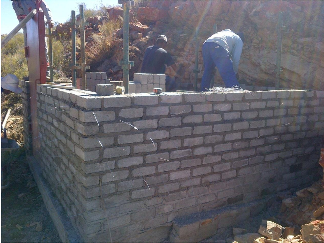
Figure C.5: Walls with installation of the steel door and wire on the outside, which holds the stone cladding to the sides.
