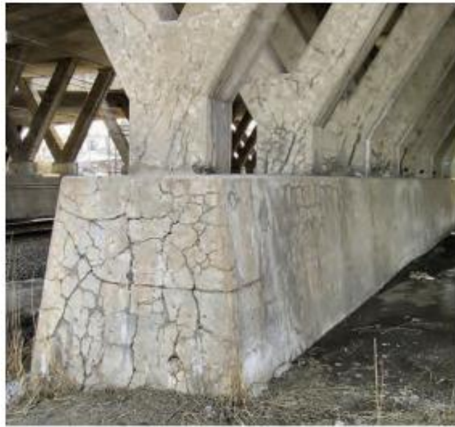
Figure 2.12: ASR in a bridge showing map cracks affecting the aesthetic value of the structure (Reactive Solutions, 2012).
