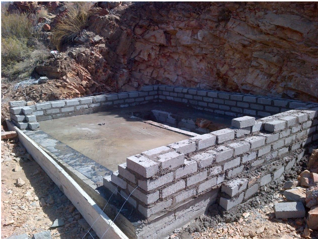
Figure C.4: Walls of the vault strengthened with 'brick force' wire.
