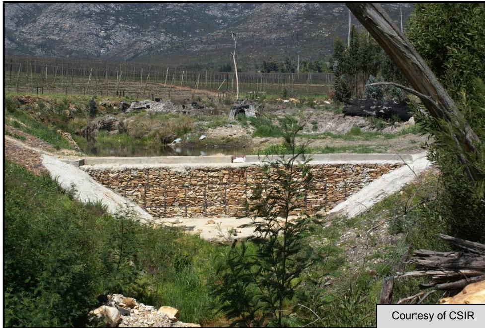
Figure 2.13: An example of a structure built in the river to rehabilitate the river channel
