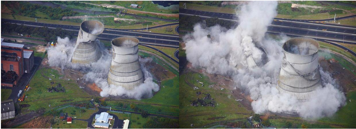
Figure 2.7 Demolition of Athlone cooling tower in 2010 by implosion (Athlone Towers Demolition (left), 2010 and Athlone Towers Demolition (right), 2010)
