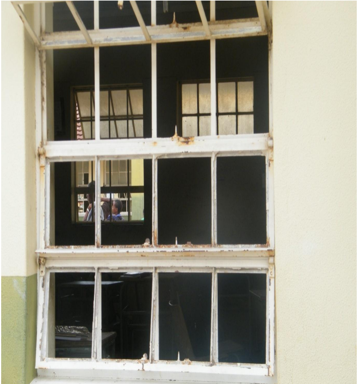
Figure 14: Condition of windows in one of the schools
