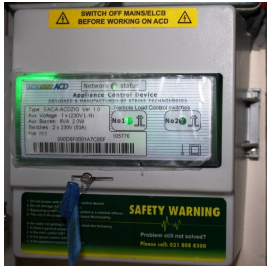
Figure C-2: Installed device to switch geyser on and off
