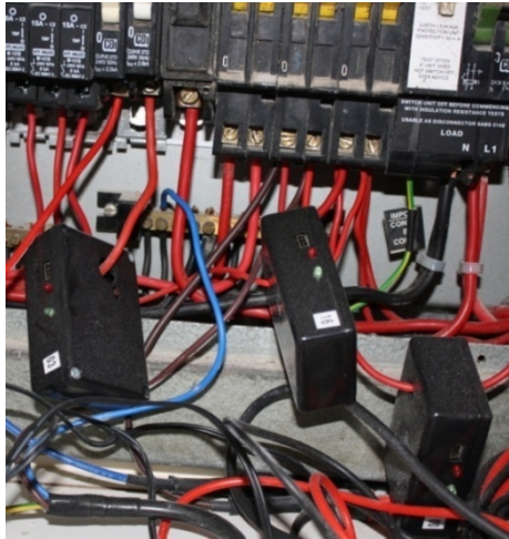
Figure 4-10: Data loggers for equipment with direct connections to the household circuit
