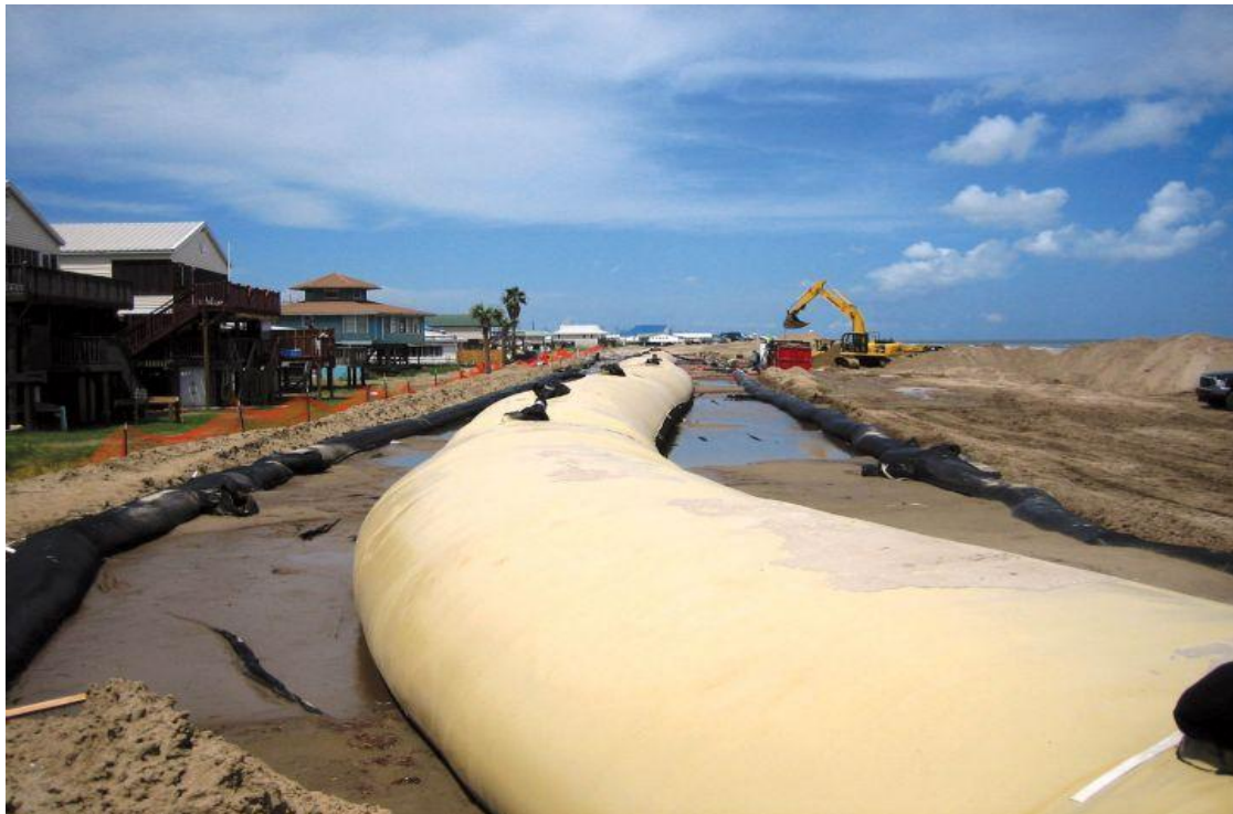
Figure 2.10: Geotextile tube as shore protection in Grand Isle, Louisiana. (Photo: TenCate Geosynthetics)
