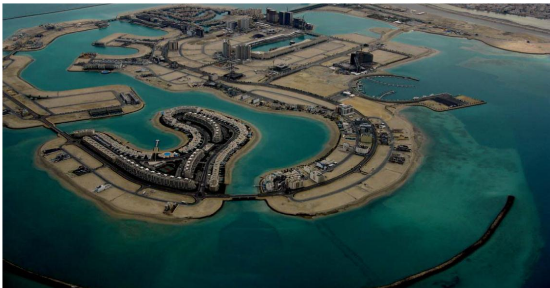
Figure 2.16: Aerial view of Amwaj Islands (photo: Ten Cate Geosynthetics)
