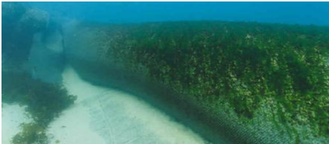
Figure 2.30: Seaweed covered submerged geotextile tube at Young-Jin beach (Oh & Shin 2006)
