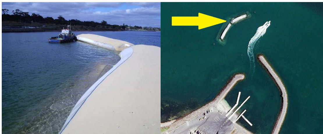
Figure 2.25: Limeburners breakwater (photo: Geofabrics Australia) (Google Earth)
