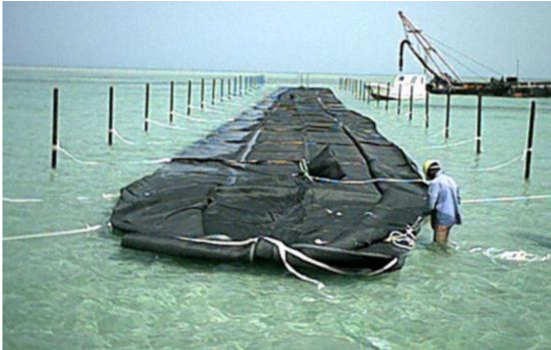
Figure 2.19: Geotube® placement before filling started. Note the fixing of the tube against horizontal movement (Fowler et al, 2002).
