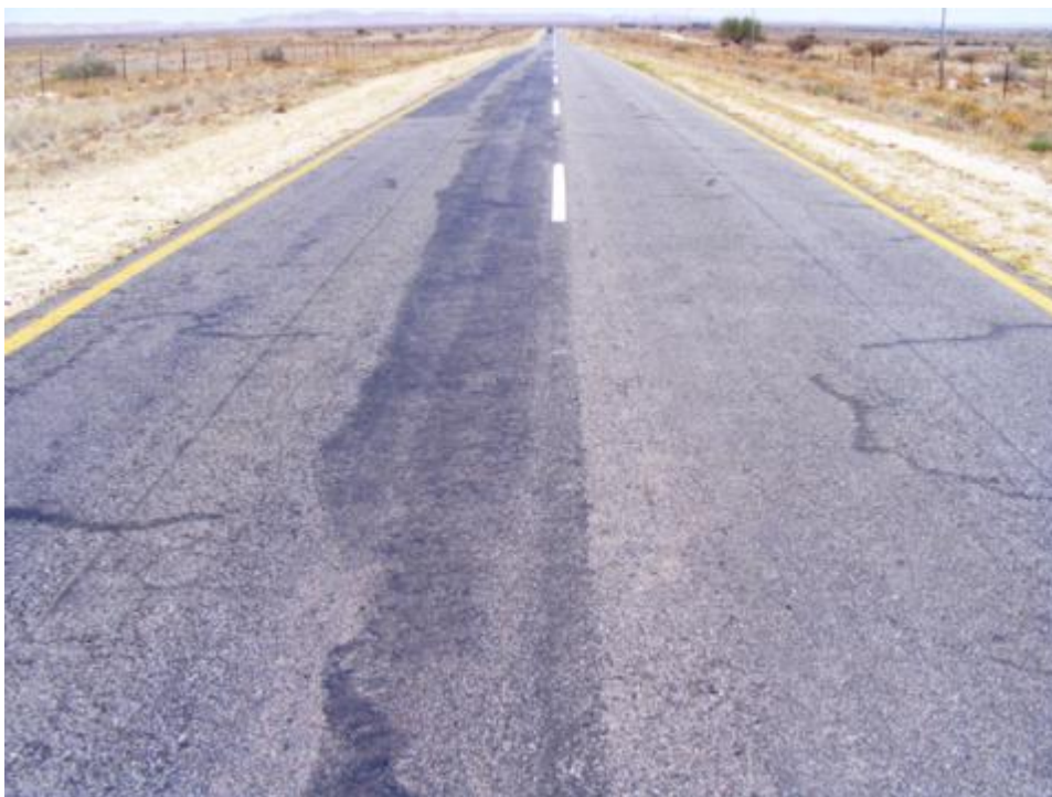
Photo 3-2- Area showing signs of bleeding
