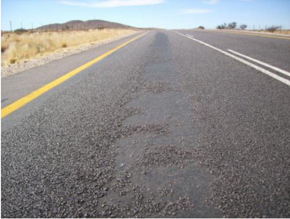
Photo 3-1- Areas showing ravelling and stone loss.
