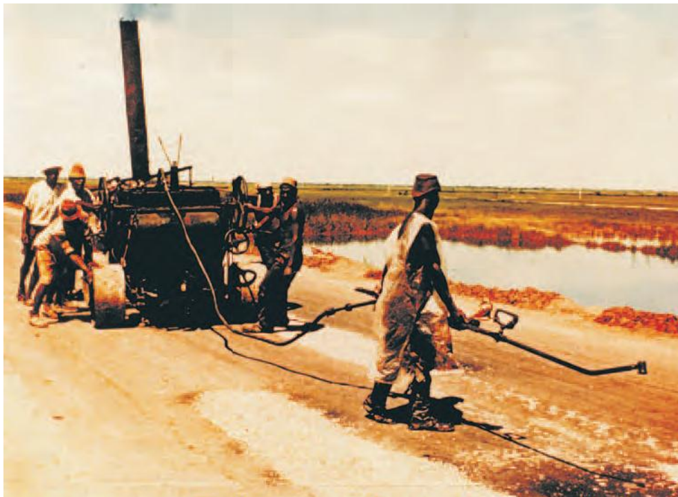
Photo 2-2- Early Bitumen Spray Operations (SABITA, 2009)
