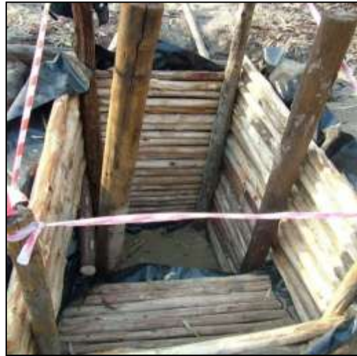
Image 3-2: Wood structure preventing soil collapsing into pit
