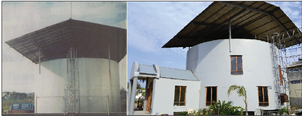
Figure 2-2: An old wine tank (left, Brümmer, [s.a.]) retrofitted and now used as a house (right).
