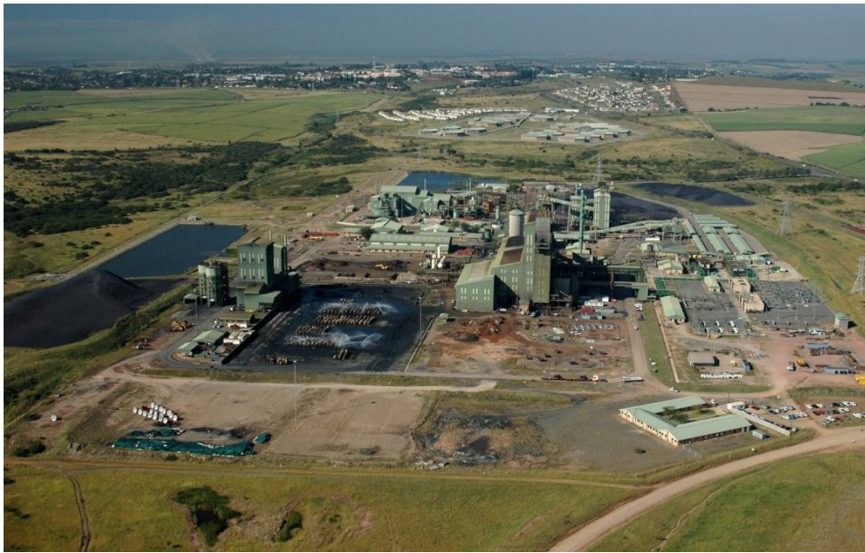
Figure 41: Northerly view the CPC outside Empangeni, South Africa.
