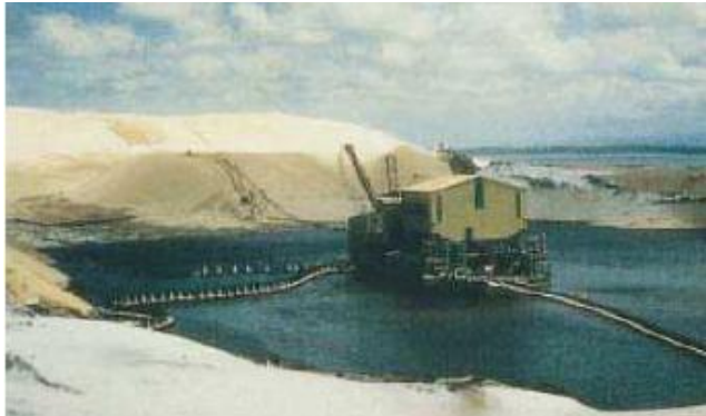
Figure 37: Dredge mining of a heavy mineral deposit
