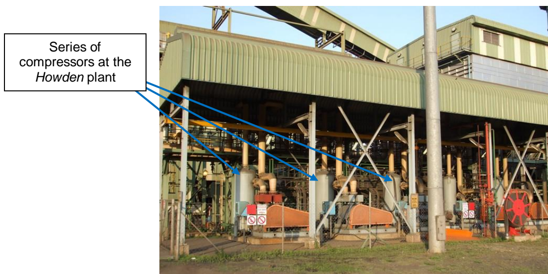
Figure 52: Howden gas compression and distribution plant
