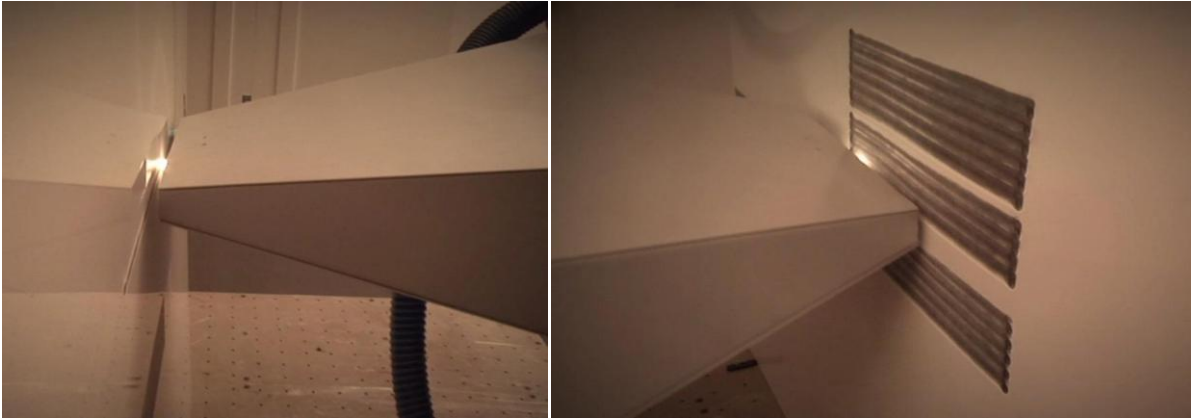
Figure 5-20 - Paint removal system in operation
