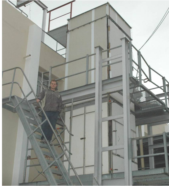
Figure 4-6: Photograph of counter-flow fill test facility.
